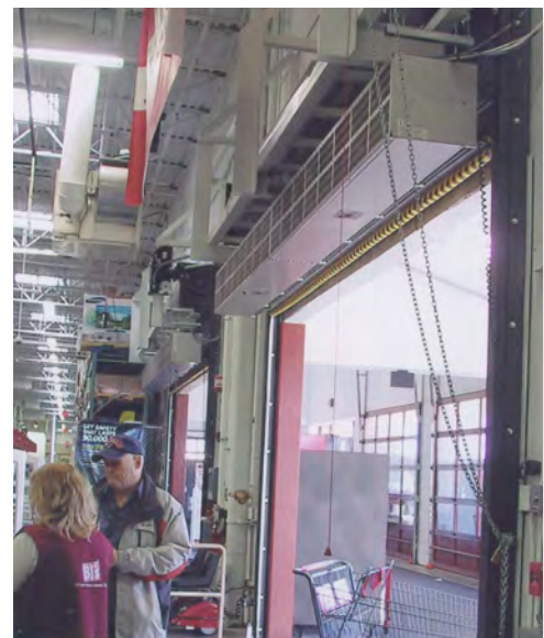
Air curtains are ideal for separating environments when physical barriers such as doors would get in the way
