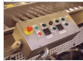
F Digital-Analog control panel
