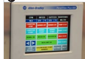
Allen Bradley PLC Control
