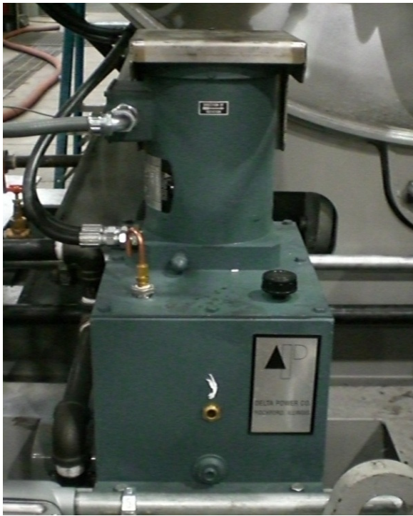
FIGURE 3-6 HYDRAULIC DOOR POWER UNIT
