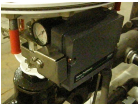
FIGURE 3-30 VALVE POSITIONER
