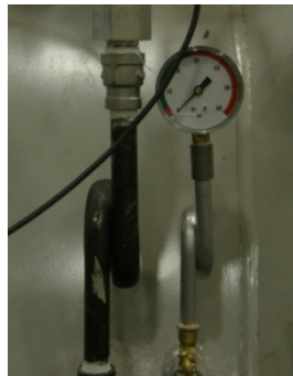
FIGURE 3-28 PRESSURE TRANS & GAUGE
