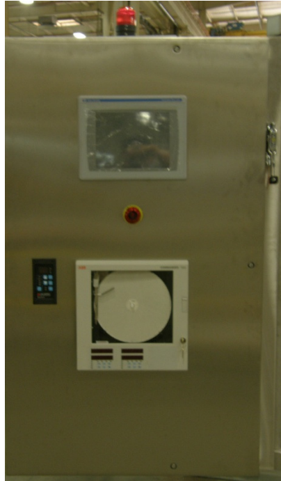
FIGURE 4-1 CONTROL PANEL WITH TOUCH SCREEN
