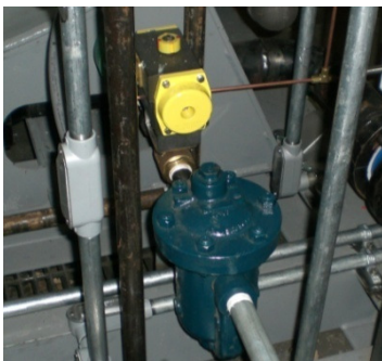
FIGURE 3-33 STEAM CONDENSATE CONTROL
