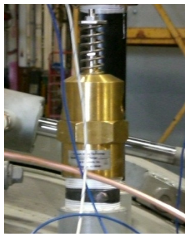
FIGURE 3-11 VACUUM BREAKER (VB1)
