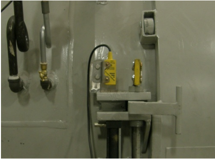
FIGURE 4-2 DOOR INTERLOCK SAFETY SWITCH
