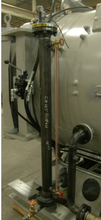
FIGURE 3-15 WATER LEVEL SIGHT GLASS
